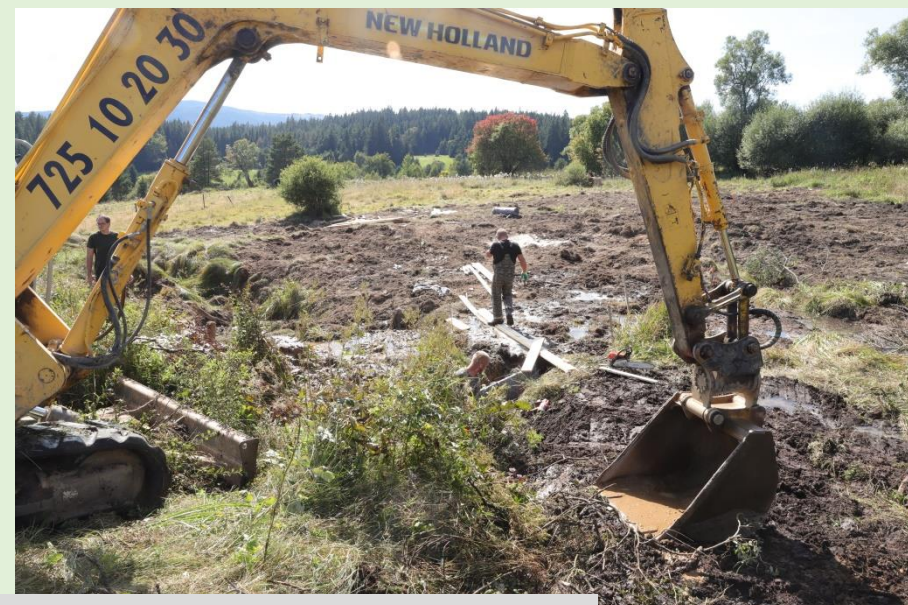
Blocking of drainage ditches, infilling of large pits from bank soil deposits
