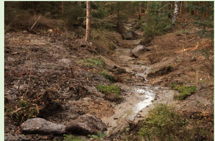
4. Increasing of stream bed and re-waving of eroded ditch (ditch was created in line of former stream)
