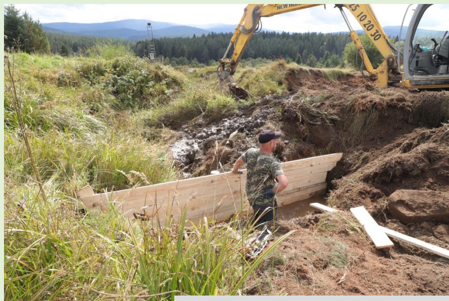
Blocking of drainage ditches, infilling of large pits from bank soil deposits
