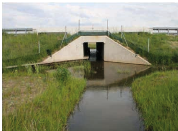
Fig. 38 Underpass for small animals permanently flooded by water 129
