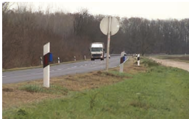
Fig. 22 Blue retro reflectors installed on odometers on Main Road 1 in Hungary, successfully reducing wildlife collisions. Area surrounding GPS: 47°50'59.4"N 17°27'00.1"E
