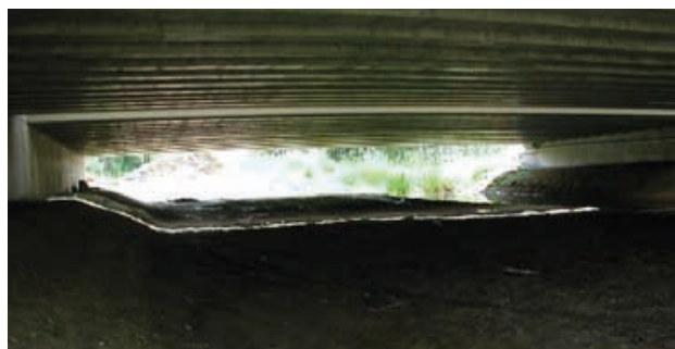
Fig. 36 Poorly implemented, too low wildlife underpass in Hungary 128
