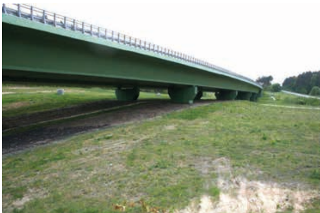
Fig. 37 S-3 expressway Międzyrzecz – Świebodzin. Viaduct for large animals close to Nietoperek in Poland, where the height is limiting the possibilities of the animals to move from one way to another.
