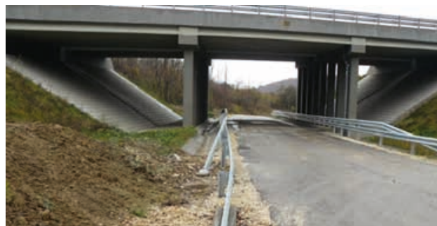
Fig. 35 Poorly implemented wildlife crossing with concrete on M7 Motorway at Kőröshegy in Hungary. GPS: 46°48'58.7"N 17°54'10.1"E 128
