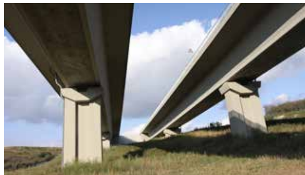
Fig. 10.35 When a viaduct has a split construction, the surface under the bridge has enough light and precipitation for the growth of vegetation. That allows for a better connection of habitats. On the other hand, the overall width of impacted area is greater compared to a unified construction, which is also true for noise intensity under the bridge. Hungary. © Václav Hlaváč
