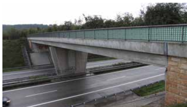
Fig. 10.30 A bridge for a forest path over a motorway was in this case widened by 2 m on each side and the new strips were planted with bushes. Disturbances are eliminated by protection walls (full railing). Such a multi-purpose overpass can be used by smaller mammal species (up to the size of fox or badger), but also by small birds, bats, tree top species, etc. Germany. © Václav Hlaváč
