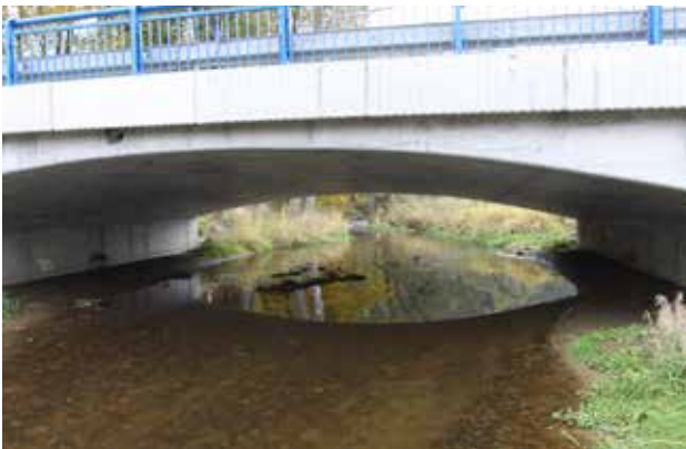
Fig. 10.8 Birds such as the common kingfisher, the white-throated dipper, or the grey wagtail are able to fly under a bridge with the openness index of at least 1-2. Height is also important; it should be minimally 2 m. In case of bridges with smaller dimensions birds typically fly over them and often become traffic victims. © Václav Hlaváč
