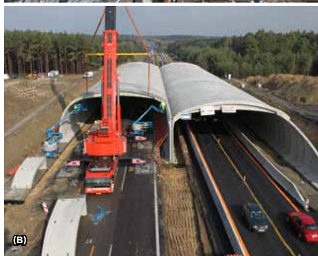
Fig. 9.16 A) Construction of the bored tunnel Višňové on motorway D1, Slovakia. B) Construction of a cut-and-cover tunnel - green bridge near Moravský Svätý Ján, Slovakia. © NDS Archive
