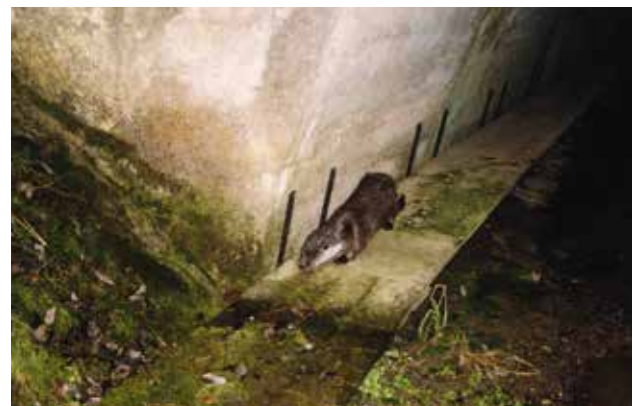
Fig. 10.13 In the case of bridges without dry banks it is possible to create additional "animal ledges." The natural continuity of the "path" to the stream banks must be maintained. © Václav Hlaváč
