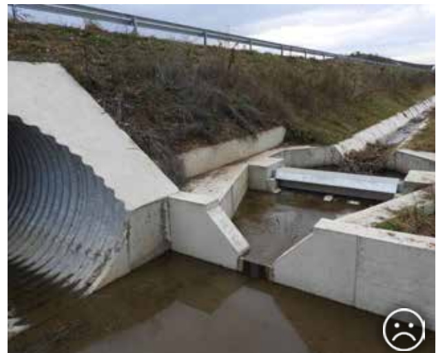
Fig. 9.18 Culverts of larger diameter should always be adapted for passage of fauna under a motorway as well. The outflow is in this case technically arranged in a way that completely eliminates the possibility to use the culvert as fauna passage. In addition, it can create a deadly trap for small animals (amphibians, small mammals) trying to pass through. © Václav Hlaváč
