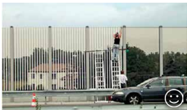
Fig. 10.60 The process of installation of glued stripes to a noise protection wall on D47 motorway in the Czech Republic. In 2008, almost 200 dead birds were found along just 1 km long stretch of this motorway between Bohumín and Ostrava within 6 months. This mortality rate dropped practically to zero after equipping the wall with the stripes. © Jan Mayer
