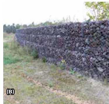
Fig. 10.28 Protection walls effectively reduce disturbances on green bridges. They can be made of wood (A), plastic, or in the form of stone walls (B). Stone walls have disadvantages in higher costs and greater load on the bridge, but also advantages in unlimited lifespan and creating new habitats (for example for reptiles).
