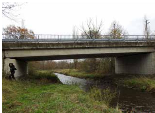
Fig. 9.9 Properly designed bridge over a stream with dry banks that allows for movement of most animal groups. © Lukáš Poledník
