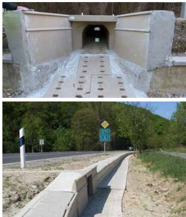
Fig. 10.48 An amphibian tunnel is a good solution for overcoming narrow roads of lower category. Barriers guiding animals to the passage are a necessary condition for proper functionality. © András Weipert
