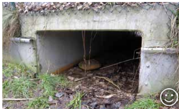
Fig. 10.43 Rectangular culvert is a good solution for amphibians, reptiles and mammals up to the size of fox or badger. © Lukáš Poledník
