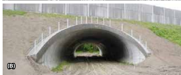
Fig. 10.37 Behaviour of animals near underpasses makes it evident that they register the noise caused by the passing vehicles (bearings of the bridge plate) - (A). Therefore, while constructing new bridges, it is always necessary to choose a solution that minimizes noise under the bridge. Noise under a bridge is best eliminated when there is a layer of soil between the bridge construction and the road/railway (B). However, this solution always brings under comparable conditions a reduction of the bridge dimensions as well. © (a) by Friends of the Earth Czech Republic, photo (b) by Nature Conservation Agency of the Czech Republic
