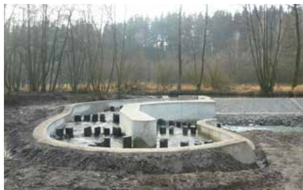
Fig. 10.49 A fish crossing in the form of a bypass – in order to overcome a weir 1.3 m high, it was necessary to create a fish crossing with a total length of 40 m. The Czech Republic. © Bohumila Jermlová
