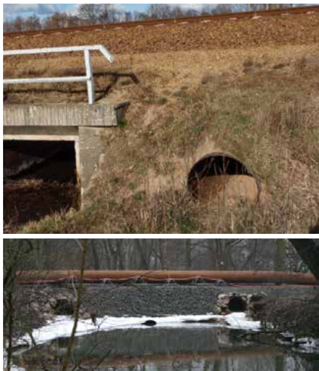
Fig. 10.47 Otter tunnels are a suitable solution in places where a bridge is impassable for otters or where transport infrastructure is led on top of a pond or reservoir dam. © Lukáš Poledník
