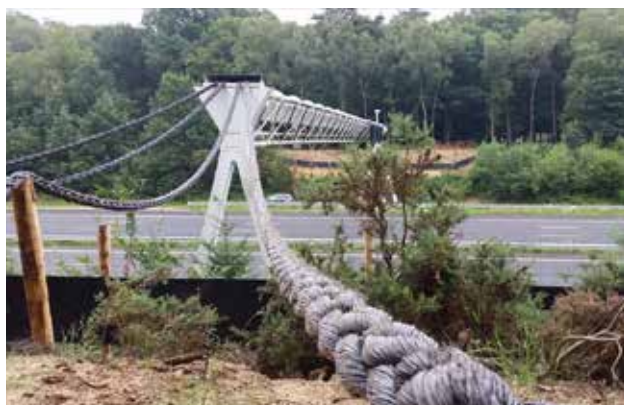
Fig. 10.16 Example of a special passage for mammals living on trees: a gantry over the A12 motorway (Utrecht - Arnhem, near Wofheze, the Netherlands) adapted for use by the pine marten. The gantry contains a "walk-path" and thick ropes connect it at both ends to the edge of the nearby forest. Use by the species has already been proven by a phototrap. © Jan Willem Burgmans, Heijmans Infra
