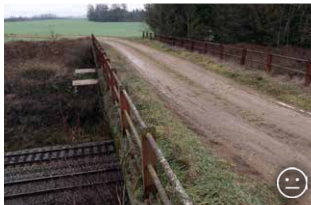
Fig. 10.2 A multi-purpose overpass over a double-track railway Prague - Brno (Czech Republic) is 7 m wide and 35 m long. Grassy stripes on the sides are used by a broad spectrum of invertebrates. Thanks to a clay surface the overpass is regularly used by the roe deer, the hare, the fox and many other species of small vertebrates, including the sand lizard. Similar bridges over motorways are used only exceptionally, because the disturbance coming from traffic is much more intense there compared to a railway. © Václav Hlaváč
