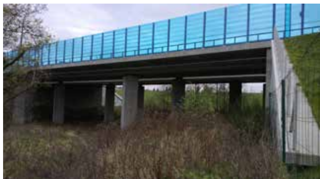
Fig. 10.38 Natural surfaces significantly improve the functionality of a wildlife underpass. A protection wall contributes to better utilization by fauna as well, thanks to disturbance elimination. A transparent wall has to be secured against bird injuries. The Czech Republic.
