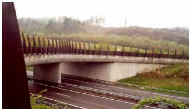
Fig. 10.24 Funnel shaped green bridge may be 40 m wide at the entrances, but only 10 m wide in the middle. This solution means financial savings without a significant influence on functionality. The picture shows the same overpass as in Fig. 10.23 in Luxembourg. © Václav Hlaváč.
