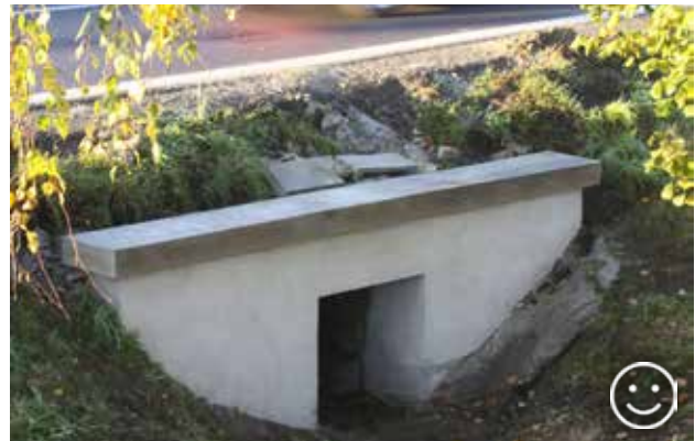
Fig. 10.4 The common toad is the most frequent target species when solving the issue of amphibian migrations over roads. Tube culverts are acceptable for this species only when there is enough light inside and the bottom is covered by washed off material. More on this topic can be found in Chapter 10.3.2.4. © Jaromír Maštera
