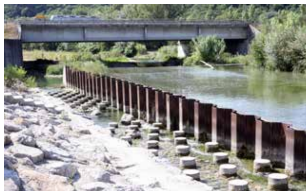
Fig. 10.50 A fish crossing near Lyon, France, where a vertical step on a watercourse was created as a result of a road construction. The fish crossing is placed directly in the watercourse and is used by the entire fish spectrum inhabiting the stream. It is also used by otters. © Václav Hlaváč
