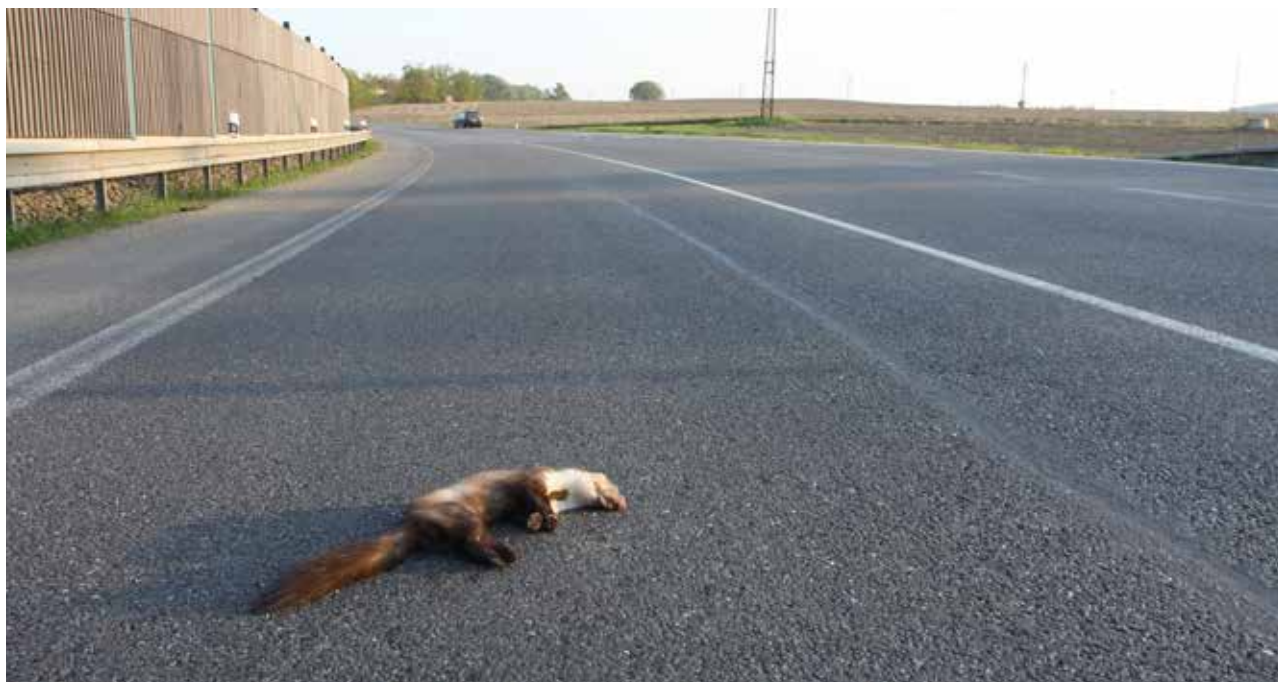
Fig. 12.10 Monitoring mortality in the Czech Republic has shown that it is very high in road sections with a noise protection wall installed only on one side of the infrastructure. Animals try to cross the road, but have to go back because of the barrier, which increases the risk of an accident. © Václav Hlaváč
