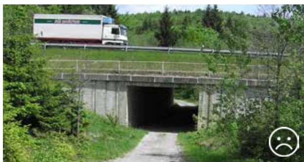
Fig. 10.40 This underpass with a forest path does not represent a suitable passage for fauna. Dimensions w = 6 m, h = 5 m, l = 33 m ( Ol = 0.9 ) are insufficient for large mammals, medium-sized mammals such as the roe deer or the wild boar use such underpasses only when disturbances are eliminated (protection wall along a motorway, limited human activities). The Czech Republic, motorway D1. © Václav Hlaváč
