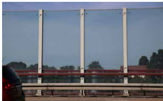
Fig. 10.61 Vertical stripes or wire mesh in glass are a reliable protection from bird injuries, they at the same time represent an acceptable solution with respect to architecture. © Václav Hlaváč
